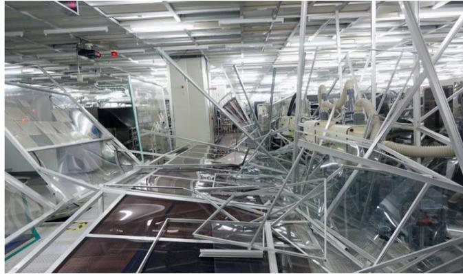
*Figure 1. Non-structural Element Failure Inside Sony's Sensory Plant [3]*
